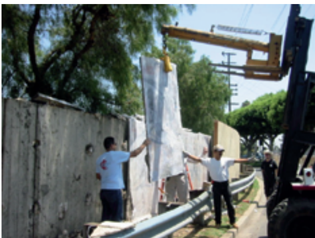
Fig. 3 De-installation of the mural, showing texture from wooden moulds on the concrete wall and plaster 'slop' on the wall.
